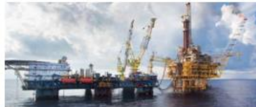
PV DRILLING V - TAD Year: 2011
